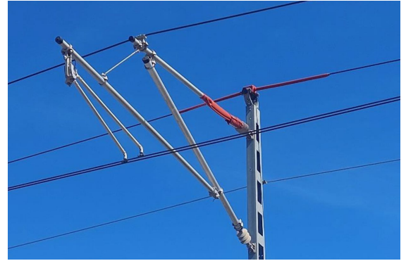
Figure 26. Correction of overhead contact line pole on Line 300 Madrid/Chamartín-Valencia
