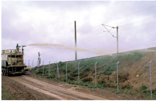
Figure 27. Fire protection measures on tracksides.
