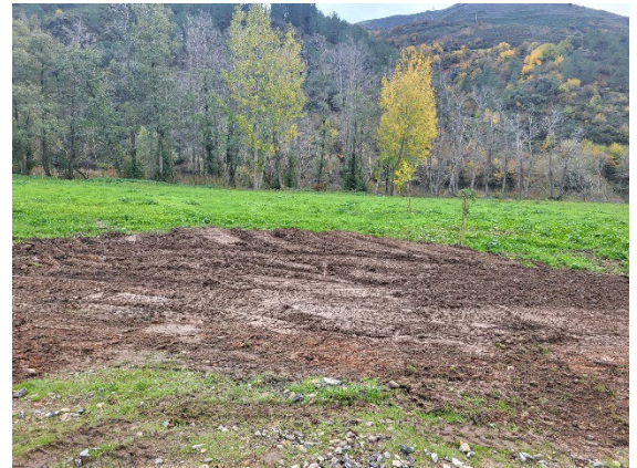
Figure 22. Backfilling of excavation pit. Ourense (environmental emergency).
