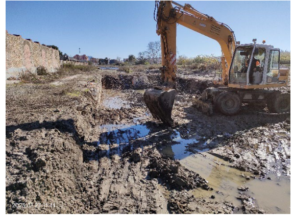
Figure 13. Soil excavation. Algeciras.
