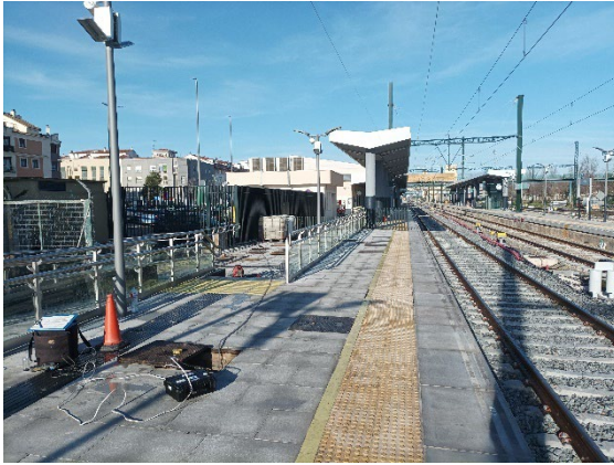
Figure 15. Level measurement. General view of the site. Badajoz.
