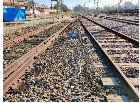
Figure 20. Purge of borehole in the rail area, Cordoba.
