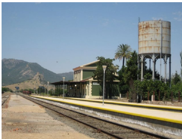
Figure 39. Almorchón Logistics Facility (Badajoz)
