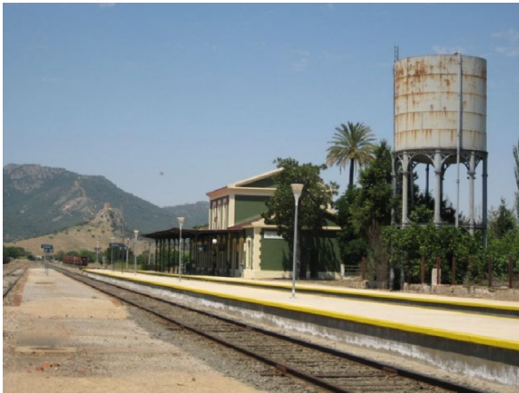
Figure 40. Almorchón Logistics Facility (Badajoz)
