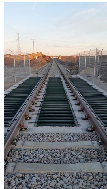
Figure 31. View of the completed Canadian crossing
