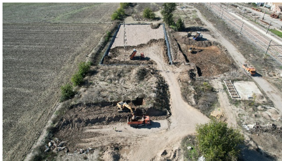
Figure 12. Landfarming preparation. Andújar
