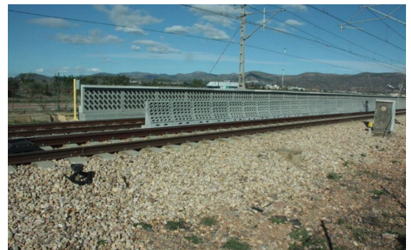
Figure 23. Testing of mini and micro acoustic barriers on the railway network
