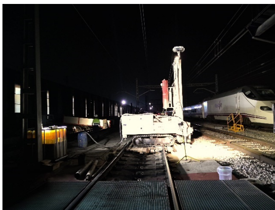
Figure 14. Conducting a night-time drilling. Fuencarral
