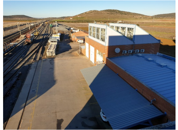
Figure 45. Calatrava High Speed Maintenance Base
