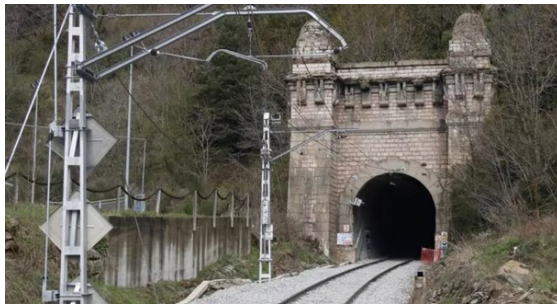
Figure 33. Recent work on the Tosés Tunnel, Gerona
