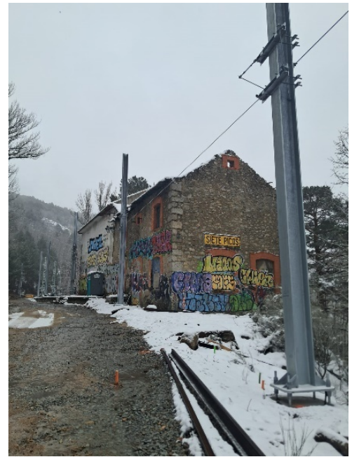
Figure 36. Work around the seven-peaked halt, a protected feature, under monitoring and control permit from the Ministry of Culture. Cercedilla-Cotos line
