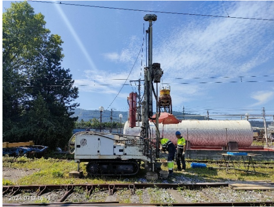
Figure 15. Drilling conduction. Irún
