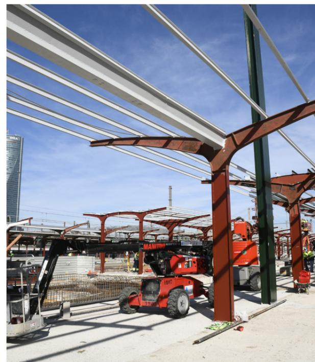
As for the north end of Chamartín Station, the remodeling project for the Iberian width tracks and platforms proposes to provide a total of 13 tracks for the Iberian width station, allowing the removal of tracks 14 and 15, their subsequent conversion to UIC standard width and their integration into the high-speed station. Likewise, the adaptation and remodeling of the respective platforms and the update of the interlocking that governs the station are also contemplated.
